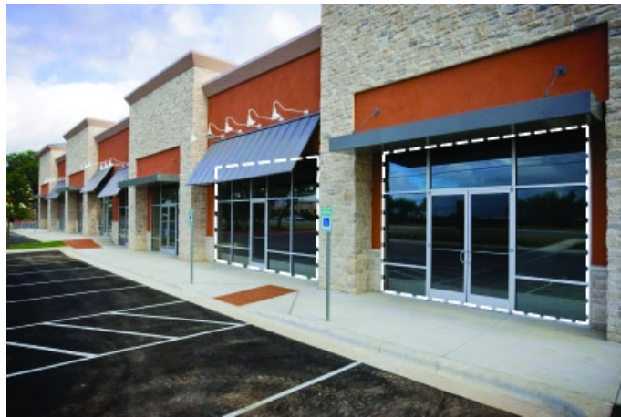
Figure G The window area is illustrated within the dashed line area for the two storefronts in the above image. The dashed lines highlight two separate window areas due to the separation by an architectural feature not related to the windows.
