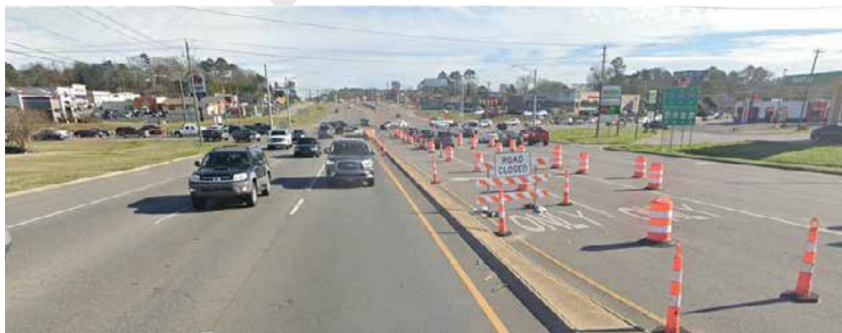
Improvements underway on McFarland Boulevard (US-82)
