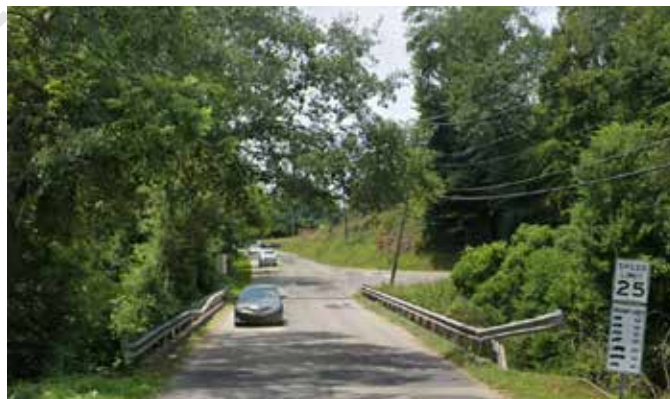
Two transportation projects are currently in design phase that will improve travel on existing roadways: Martin Luther King Jr Boulevard (including replacement of the bridge shown above) and US-43 from Mitt Lary Road to Paul Howell Road.
