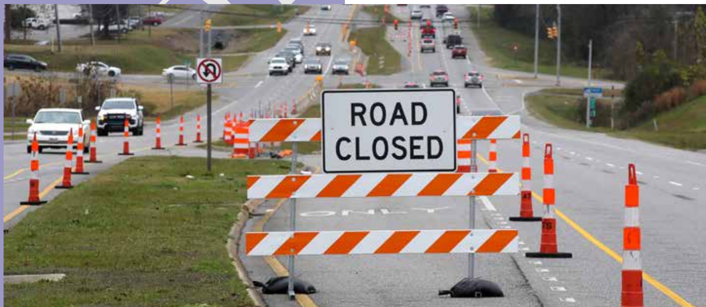
Work on McFarland Boulevard to improve traffic flow was underway during development of the Comprehensive Plan
