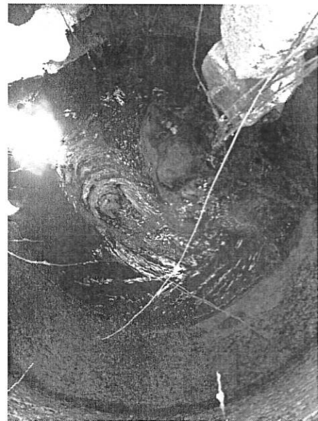
Photo 1.03B: Trunk Line Manhole
