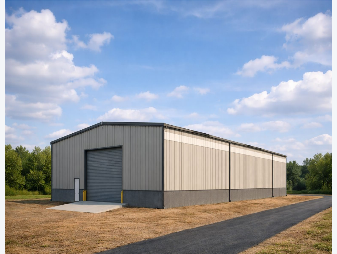
Dedicated covered staging for mill expansion components
